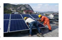
back sheet or other broken part of the module. Please install with dry tools in dry condition. Do not operate when the module is wet, unless wear proper equipment against electrical shock. Do not grab the PV module at only one side, the frame may bend. Grab the PV module at two sides facing each other. Do not touch the PV module with bare hands. The frame of PV module has sharp edges and may cause injury.
