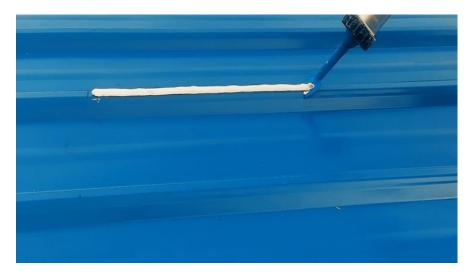
The glue length L2 is the same at the width of PV panel, distance between glue L1 should be less than 520mm, If module hanging part is above 50mm, use Aluminum support rail.
