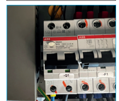
Fig. 05: Line/fault-current circuit breaker and load-break switch
