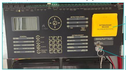
Press the extinguishant release button under the yellow cover for manually suppressing fire.
