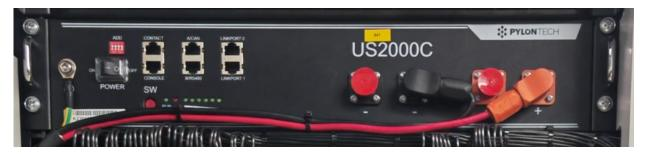
Turn on the Power switch of US2000C. Press the "SW" button of US2000C for about 3 seconds, and observe the indicator light of the UPS host. If there is mains power, the indicator light is green, indicating normal startup.
