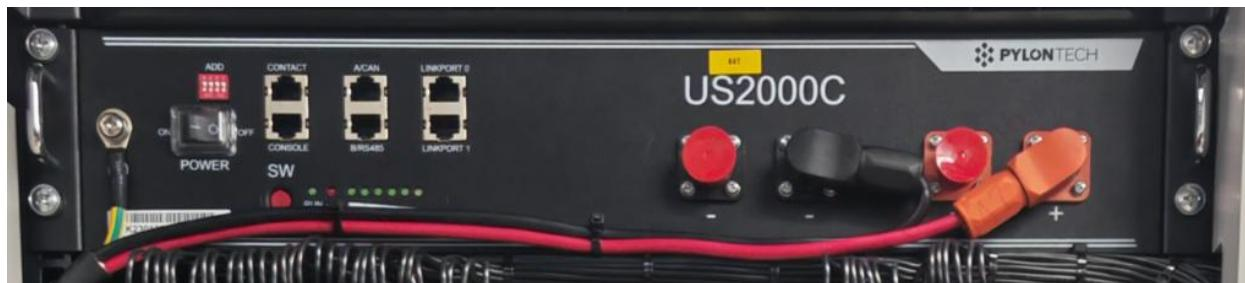
Turn on the Power switch of US2000C. Press the "SW" button of US2000C for about 3 seconds, and observe the indicator light of the UPS host. If there is mains power, the indicator light is green, indicating normal startup.
