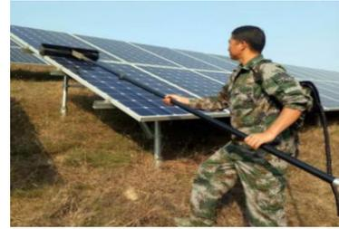
During operation of modules, there shall be no environmental factors to shade modules fully or partially. These environment factors including other modules, module mounting system, birds dwelling, dust, soil or plants. These will significantly reduce output power. EGing suggests that the module surface should not be shadowed in any case. Frequency of cleaning depends on dirt accumulation speed. In normal situations, rainwater will clean the module surface and reduce the cleaning frequency.
